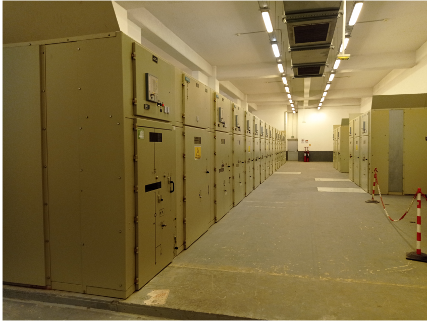
Figure 2.4: Arrival and traction bridges.
