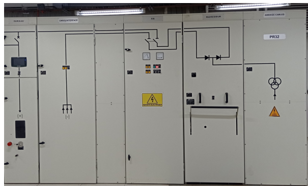
Figure 2.9: Transformer rectifier.
