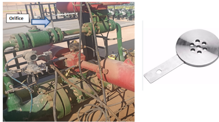
Figure A.18 : Orifice de restriction
