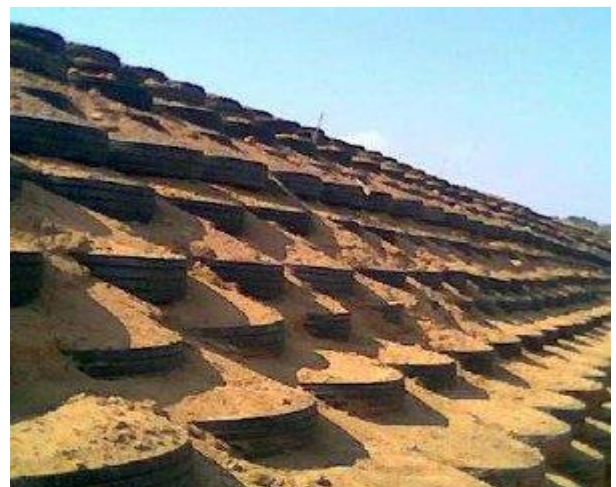
Figure 1-34 la technique pneusol á Bou-smail [38]
